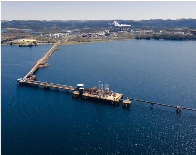
Braya, Renewable Diesel Refinery, Canada
